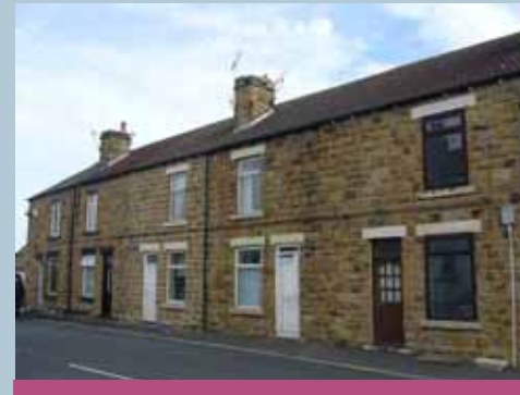
Simply detailed 19th century industrial workers terraces
