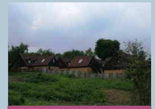
Mix of contemporary timber framed dwellings at New Farmers Hill
