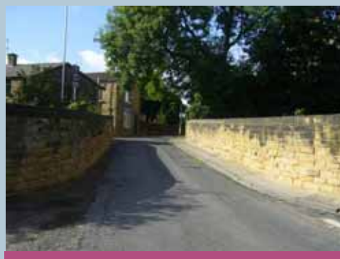
The sandstone bridge crossing the railway at Pottery Lane forms a focal point in the streetscape,
