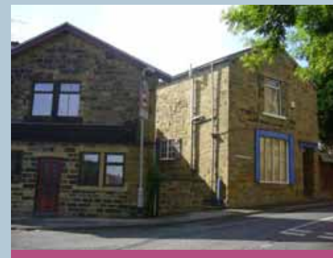
Traces of the former village shopfronts survive, Station Lane
