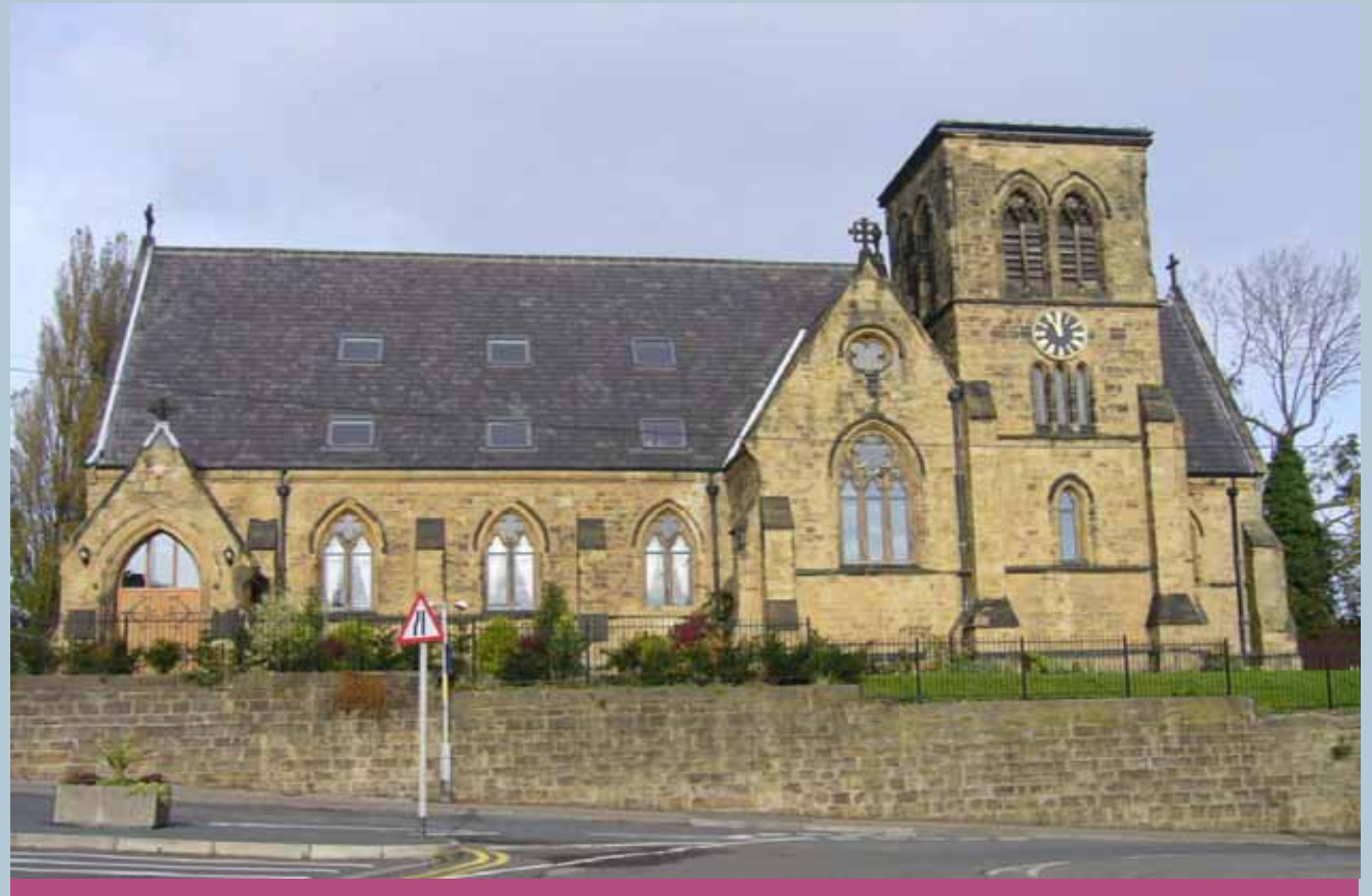
The church remains a landmark building, but the loss of its spire has weakened its impact
