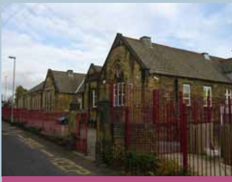
The village school opened in 1879-80 and remains in its original use today
