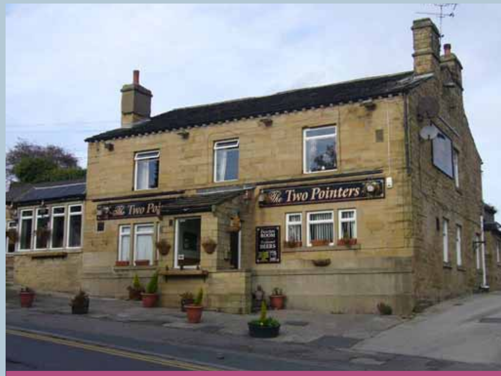
Local sandstone is a common building material. Here at Church Lane it is used as fine ashlar to the front elevation and faced, squared and coursed masonry to the side elevation
