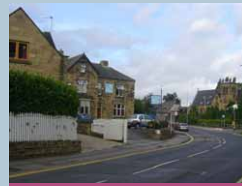
The original centre of the village is dominated by sandstone buildings
